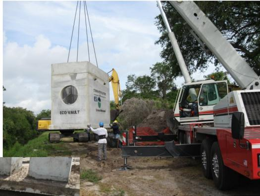
Technology is based on slowing the flow's velocity to facilitate settling.
