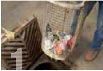
1 Remove and empty debris basket.
