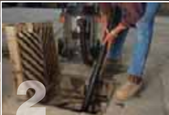
2 Clean the platform of any sediment.
