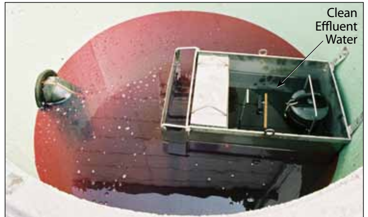
ecoLine™-b in operation with heavy oil loading on water surface
