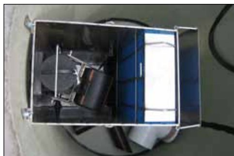
ecoLine™-b coalescing outlet structure with automatic shutoff valve
