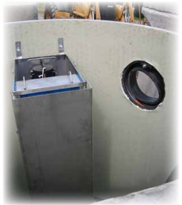
ecoLine™-b coalescing unit installed inside a lined precast concrete structure
