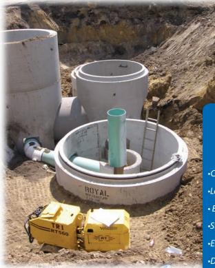
ecoStorm<sup>®</sup> design allows for tight angles between the inlet and outlet pipe. This is especially beneficial for minimizing the footprint in offline systems.
