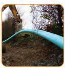
With PVC's proven long service life, Fusible Brute (CIOD) and Fusible Series (IPS) pipes are available in sizes ranging from 100mm (4") to 900mm (36") with larger sizes in development. The proprietary PVC formulation, fusion process as well as our licensing and training program allow for the consistent, reliable fusion of Fusible Brute and Fusible Series pipes to create piping systems of unparalleled strength.
