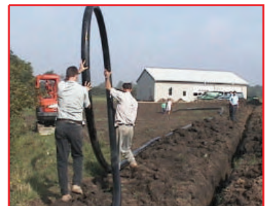
9 • PEX Flex installation
