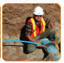
Blue904 is fully certified, lightweight and flexible PEX water service tubing. Installation friendly, Blue904 will resist corrosion, maximizing water flow over the lifetime of the system. Made with a copper tube size (CTS) OD (SDR 9), Blue904 works with standard compression fittings and is available in 3/4", 1", 1-1/4", 1-1/2" and 2" sizes.
